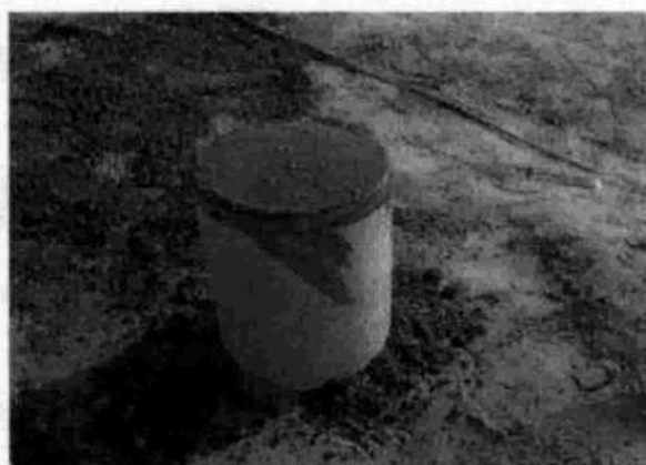
Step viii): Sealing of construction well using concrete cement material
